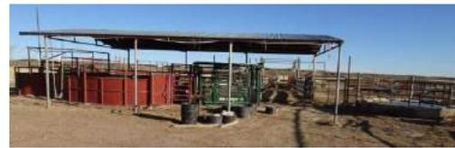
\*Malpais Well---90 feet deep with a 40 foot water level and a solar pump (6 gallon/minute). Also has a 15,000 gallon fiberglass lined storage and two 1000 gallon drinkers.
